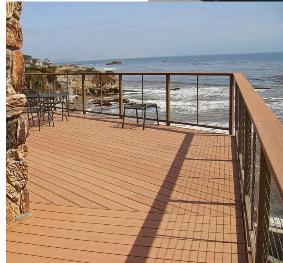
CableRail Infill Photographer: Lightworks | Installer: Moore Construction
