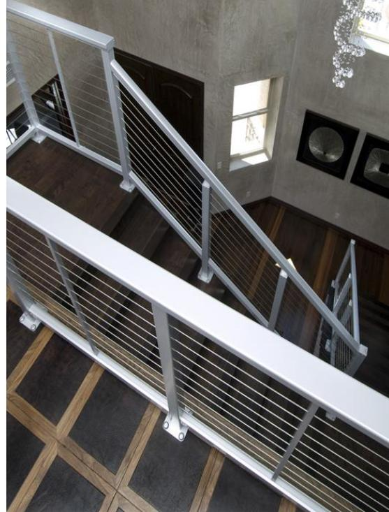
DesignRail® railings showcased on the front entry stairway of the NextGen demonstration home. The railings have a series 200 rectangular cap rail with a silver powder-coated finish and 1/8" diameter stainless steel CableRail infill cables.
