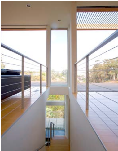
Example of the use of cable railing in residential construction. Source: Safdie Rabines Architects. Photo Credit: Adam Butler.
