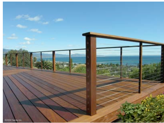
Photo of exterior deck with wood railings and CableRail
